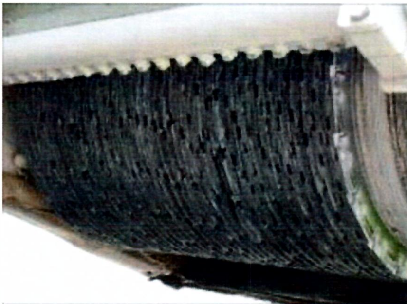
figure A6-8.Diamond grinding of cement concrete
