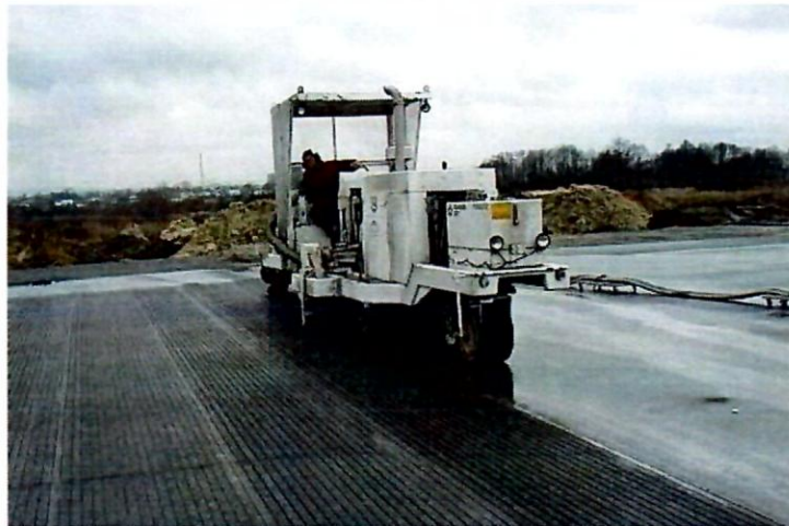
Figure A6-5. Grooving with saws
